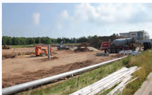
Baseball stadium progress to date
