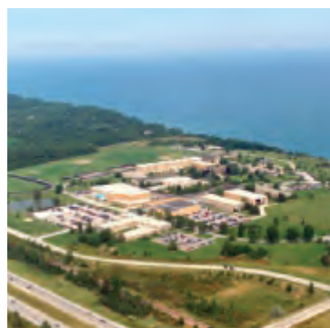
Aerial view of the Mequon campus (1981–1990).
